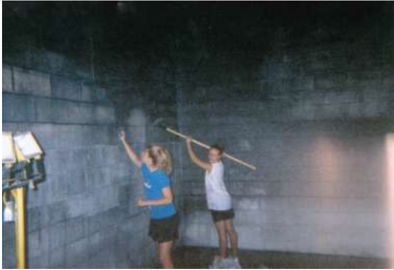
DANA SCHEFFEN AND BREANNA DETTMAN CLEANING FIRE DAMAGED SHELTER
