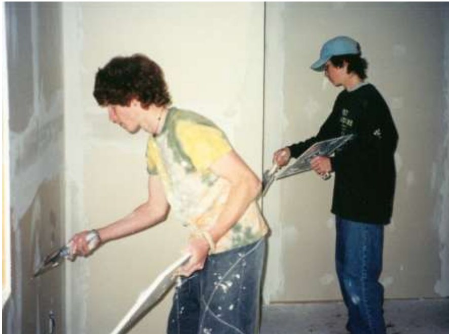
James Weber and Alex Lane finishing drywall for home
